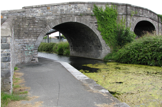
Figure 7: Royal Canal and Bridge.
